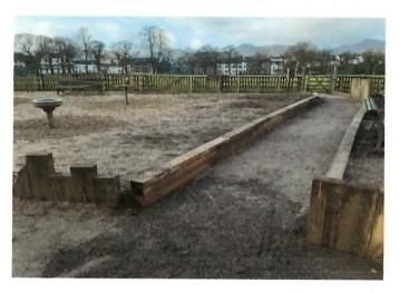
Old and rotting timbers have been replaced using some of the oak timber reclaimed from the felled oak trees within the parks. The timbers have been fixed to a new concrete foundation in time as budgets allow the path will be paved to replace the grey dust surface.
