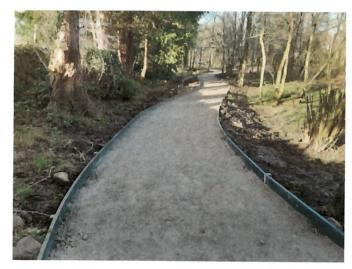
installed, recycled plastic edging boards have used to retain the path edges and the stream has cleaned out.
