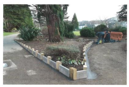
A new edge has been constructed from sleepers and paving slabs around the weeping sequoia tree. This is to prevent bark mulch creeping onto the path and help with erosion.
