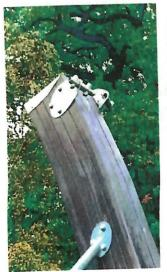
However, the damage to the cableway in the play area is far more of a concern. The cable and fixings at one end of the cableway has been damaged beyond repair and requires several new parts. This is not general wear and tear of the equipment but a deliberate attempt to damage the cableway and it will be out of action for some weeks. Two brackets and the stop spring have been damaged
