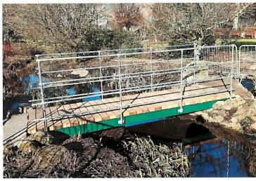
Three steel girders at 5.4 metres long have been installed to replace the wooden sleepers, the oak foot boards reinstated and a handrail made to fit to the bridge. The installation has been carried out by parks staff and brackets to secure the hand rails to the steel girders made by a local tradesman. The bridge can now be used by the public for the upcoming season.
