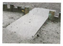
to allow space for a disabled access ramp to be installed. The existing wooden sleepers had been in place since the play area was built in 2010 and have been replaced with new sleepers.
