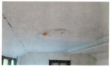
A local roofing contractor has been to look at the building and is providing a quote for the repair work. This is to replace the wooden strusses and rotting timber where required, remove and install new roofing boards and re-felt the roof. The quote will be available at the Trust meeting
