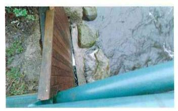
Wivell Bridge is showing the signs of water damage. The stone foundations put in after storm Desmond have moved through this winter. A licence will have to be obtained from the Environment Agency to carry out the repair work next summer. Again this is another additional cost that has to be considered.
