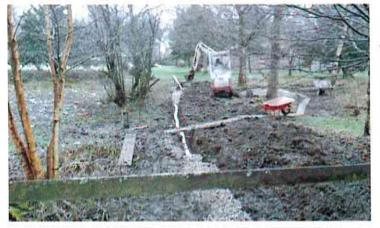
The roof/surface water drain has been dug and extended rather further than the original plans; it made sense to extend it and in order to get water away from the new buildings as far as possible.
