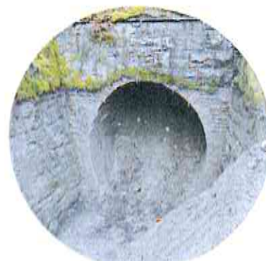
View of the existing tunnel currently packed loosely with earth
