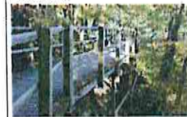
5 Boardwalk Undercutting of the bank below is threatening the stability of the boardwalk.
