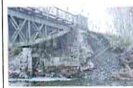
5 Boardwalk Undercutting of the bank below is threatening the stability of the boardwalk.
