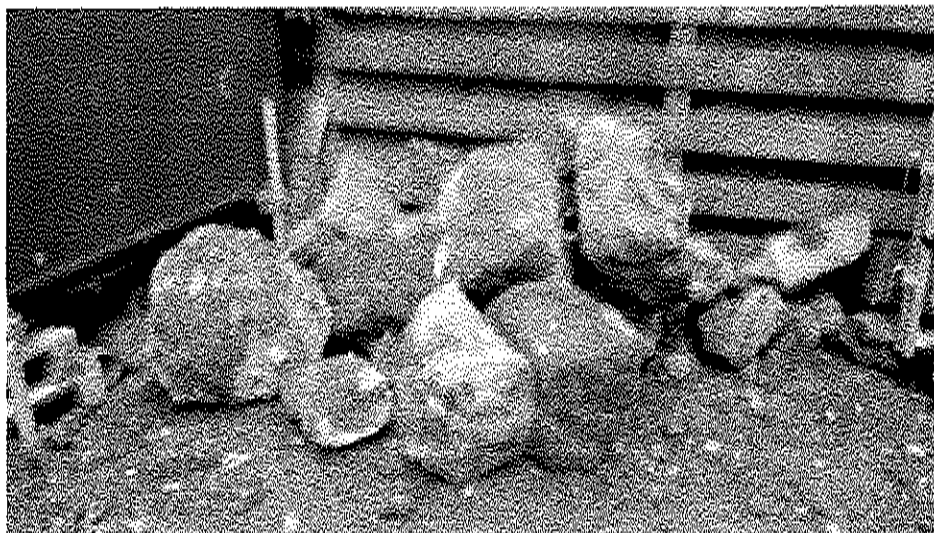
More of the concrete we have removed
